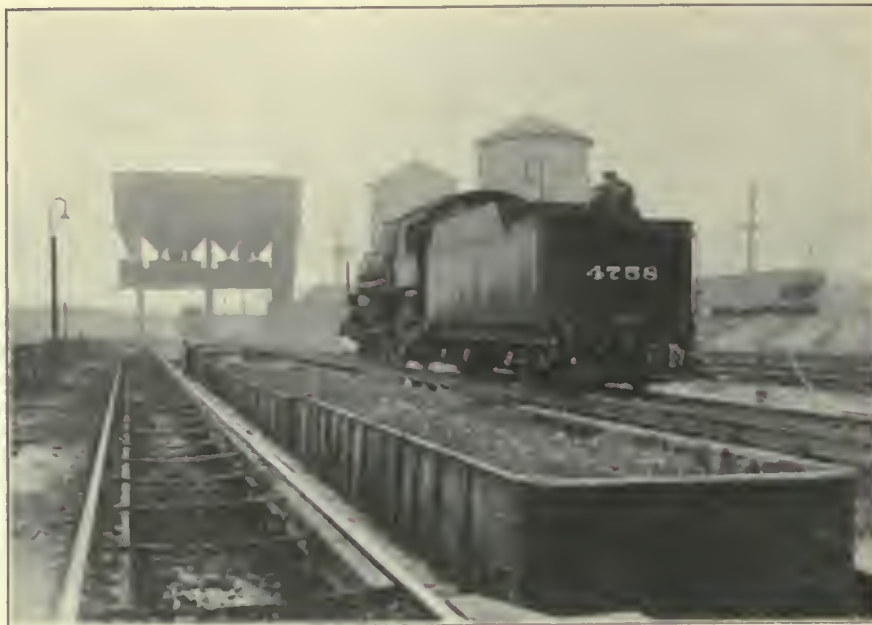
FIG. 653. FACILITIES TO BE ABANDONED. Locomotive ash-pit of the Lake Shore & Michigan Southern Railway, near 63d Street and Indiana Avenue. This is a double pit 180 feet long and is a good example of a high-class shovel-pit. The salvage of a pit of this type is very small.
